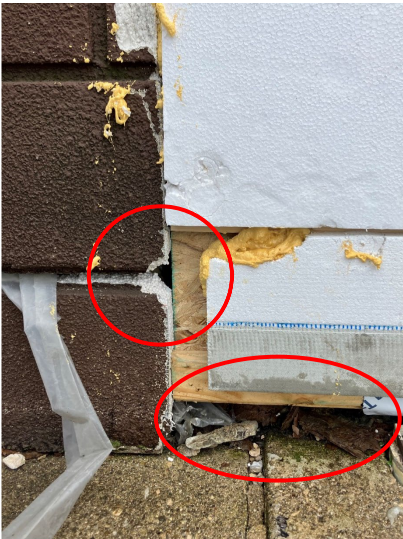
Evidence of rats/pests chewing through the styrofoam on the walls of the facility and the wood framing doesn't extend all the way to the ground, leaving room for pests to get in. These are the most recent pictures of the repairs made to the facility.
