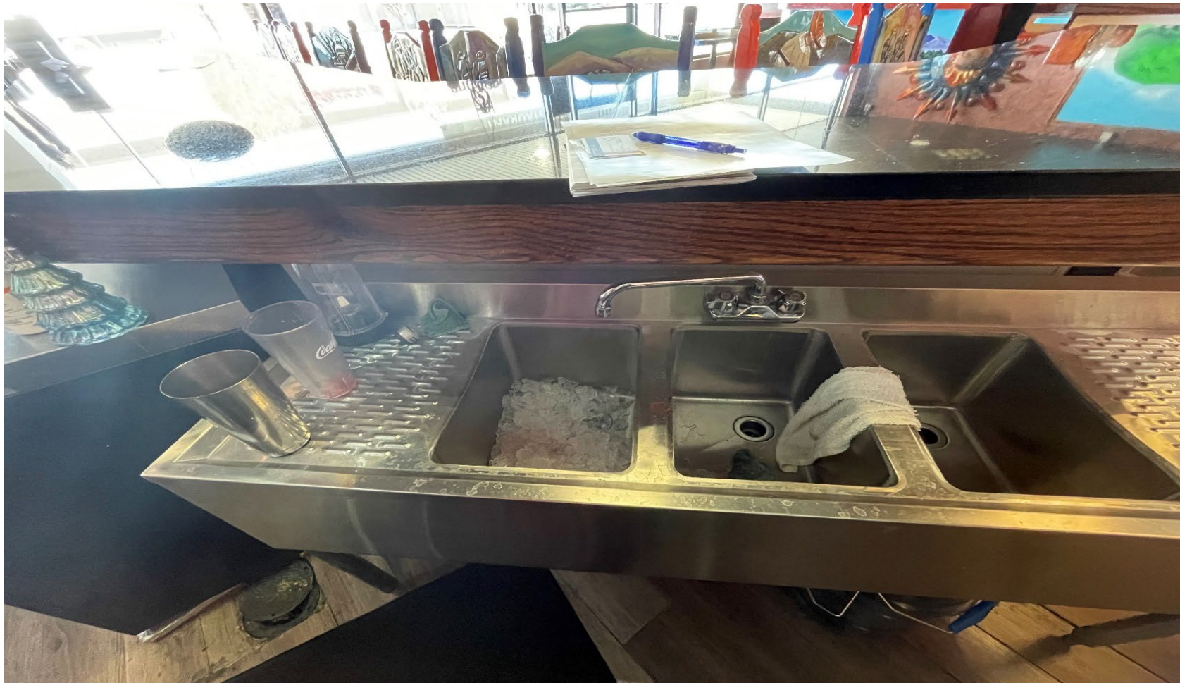
2. Photo taken 11/14/2023 at 12.56 pm. Sign of dumping ice, wet wiping cloth being stored after wiping off surfaces, used glasses and blender cup was being stored on the side of the 3-compartment sink at the bar area.
